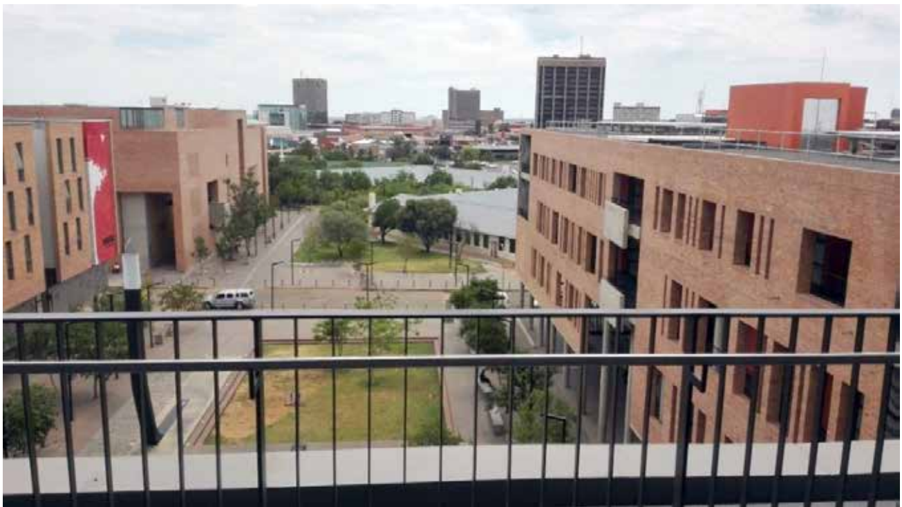
Looking at completed Central Campus Buildings from the Library
