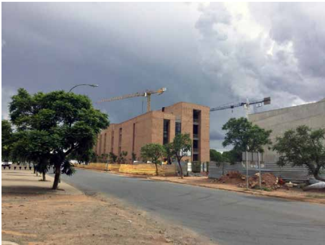
The North and East façades of the NAS Laboratory Building from Bishops Road
