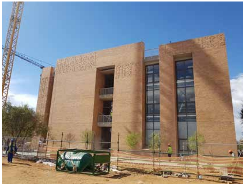
South Façade of NAS Laboratory Building
