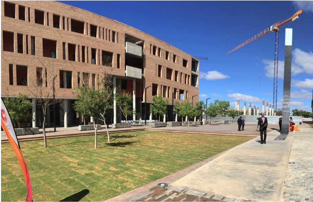
Building C003 viewed from Central Campus Square
